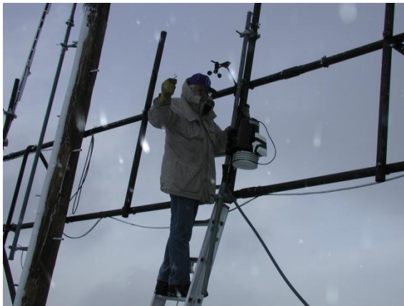
Davis Sensor Package Installation
